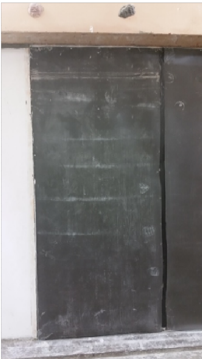
Figure 4 – Mass loaded vinyl layer installed
