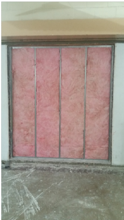
Figure 2 – Framing members and cavity insulation installed
