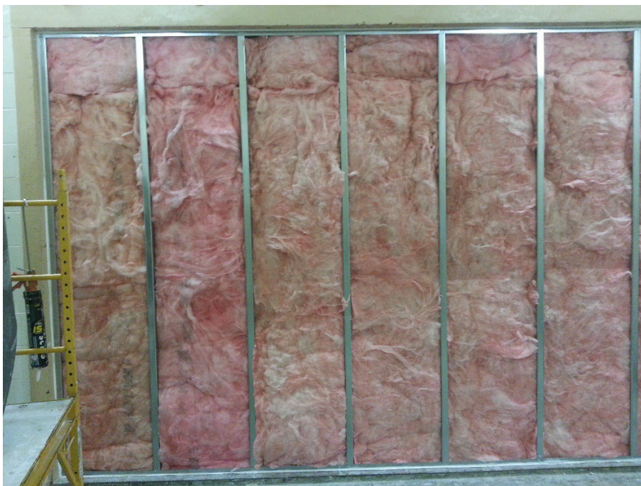
Figure 4 - Detail of insulation.
