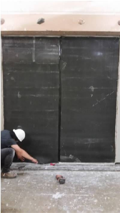
Figure 3 – Wall Blokker layer installed
