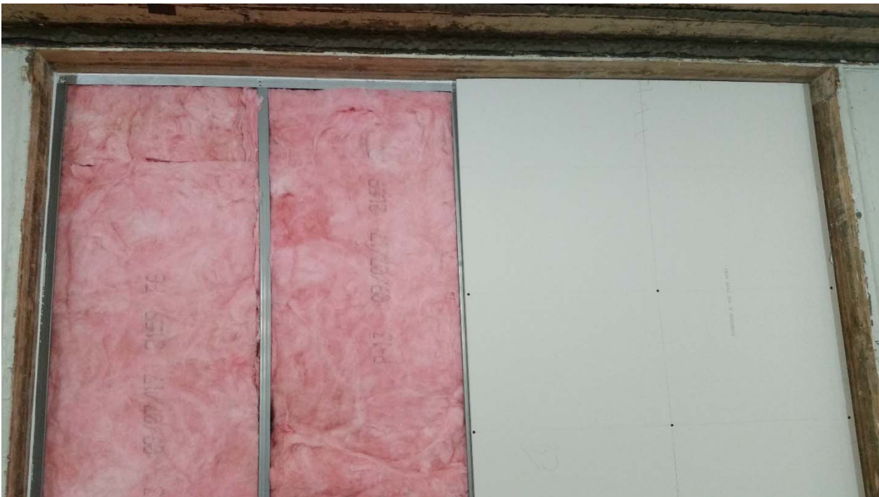
Figure 4 – Stud cavity insulation installed, receive side gypsum board partially installed
