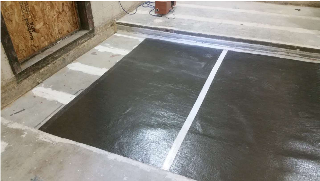
Figure 2 – Underlayment partially installed on concrete slab
