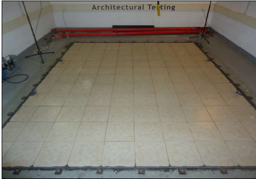
Source Room View of Test Specimen Installation
