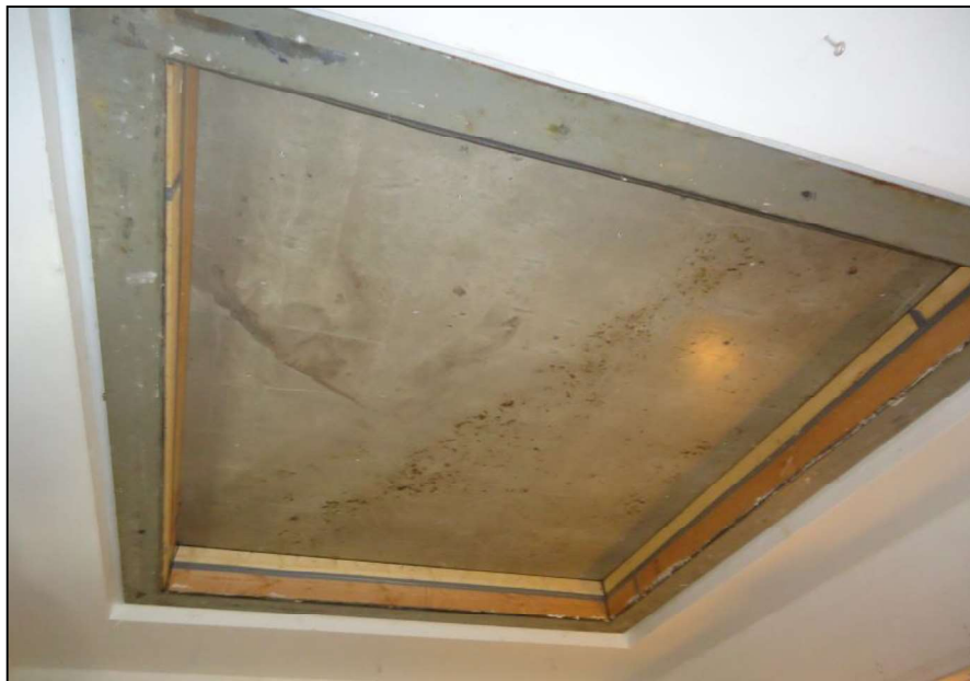
Receive Room View of Test Specimen Installation
