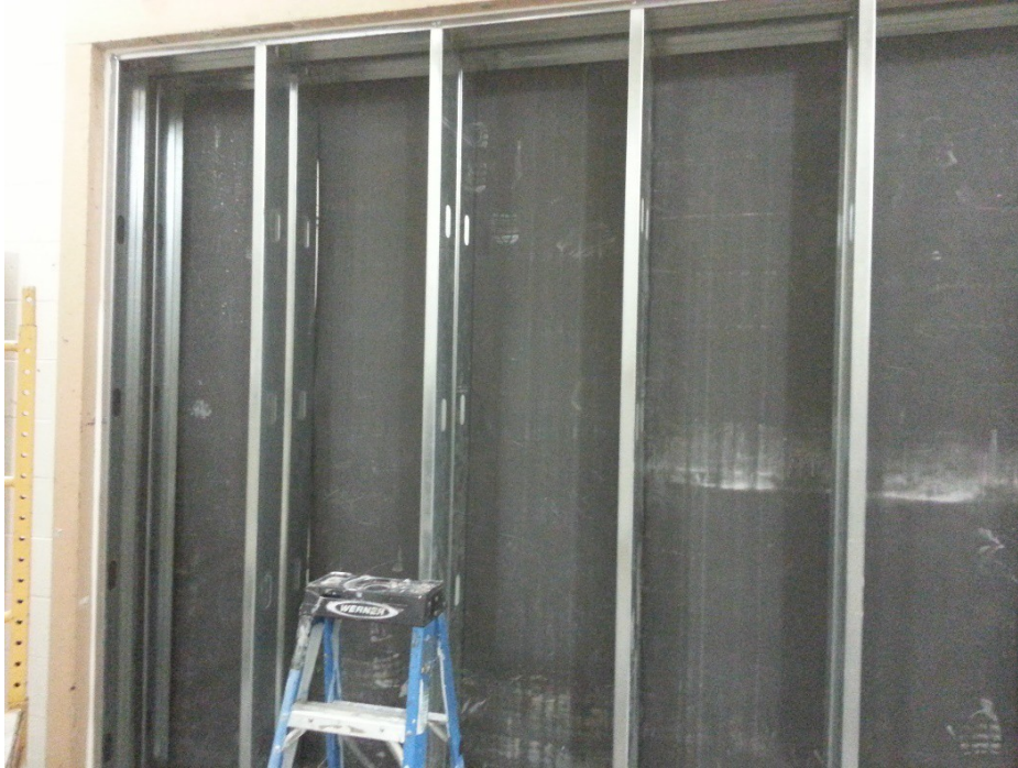
Figure 3 – Detail of studs and Wall Blokker installed on studs on one side.
