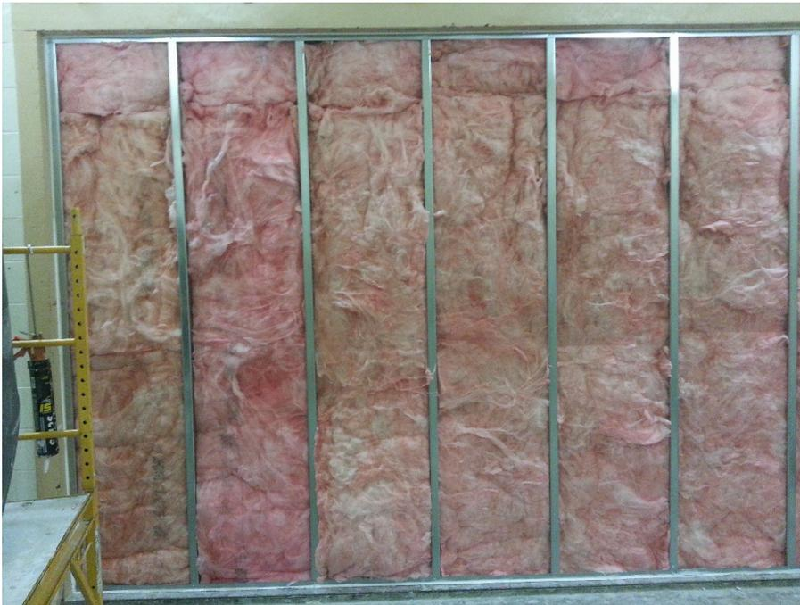
Figure 4 - Detail of insulation.
