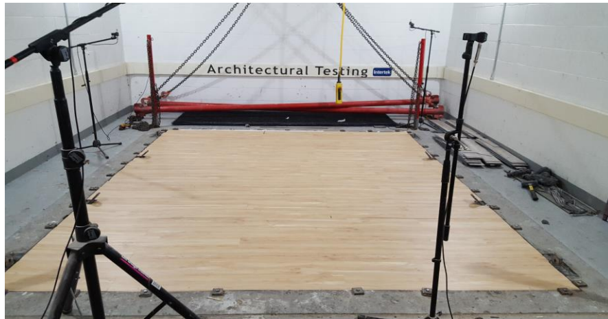
Source Room View of Test Specimen Installation
