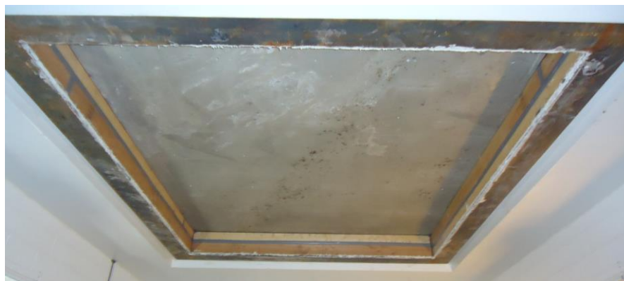
Receive Room View of Test Specimen Installation
